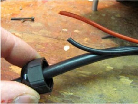
Figure 12. Thread the two 12" black and red cords through wire nut.
