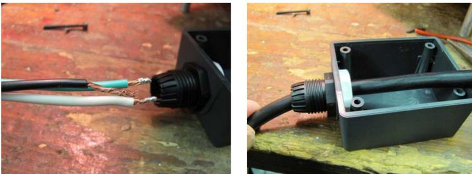
Figure 10. Thread power cord through junction box hole.
