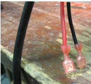
Figure 20. Crimp spade connectors onto wires.
