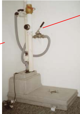
Guzzler pump operates backup sewage system in emergency shelter.
