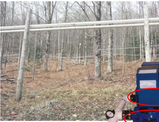
OEM sap vacuum system uses twin Guzzler GE-2600A pumps
